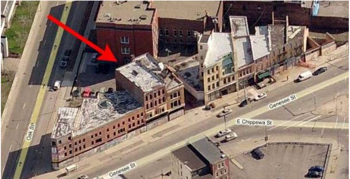
(3) Aerial View, facing south Note the regular, continuous line of the Genesee Gateway facades along the south side of Genesee Street. The Schwinn-Mandel Building is one of the most regular in mass and form compared to the other more oddly angled buildings.
