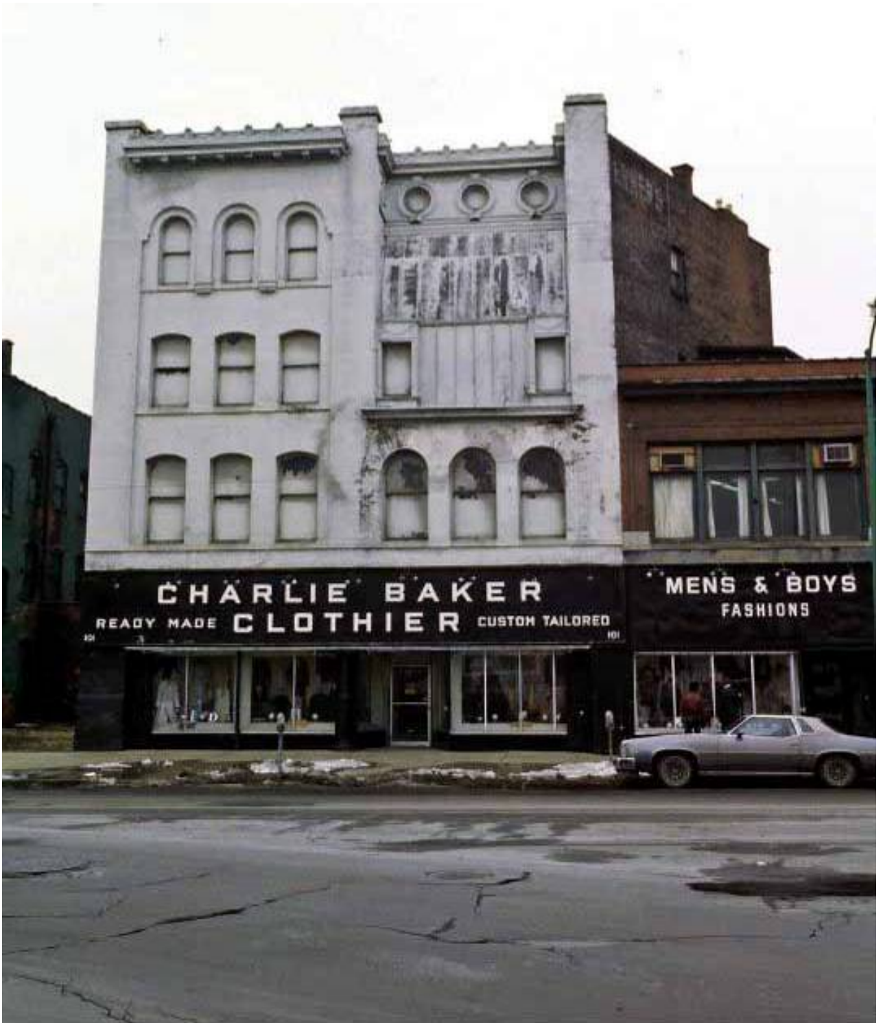
(8) The Werner Photography Building, ca. 1986
