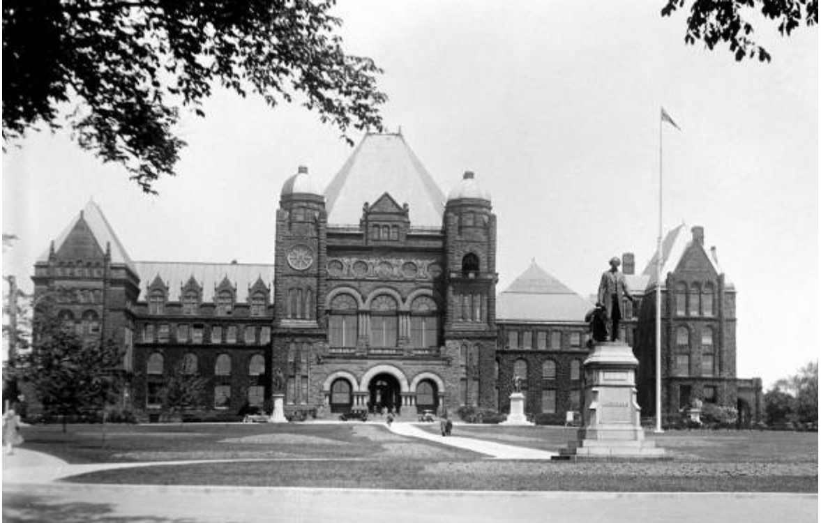
(15) Ontario Parliament Buildings (Queen's Park, Toronto) Richard A. Waite (1886-1892) A substantial extant public building which shows Waite's mastery of the Richardson Romanesque style.
