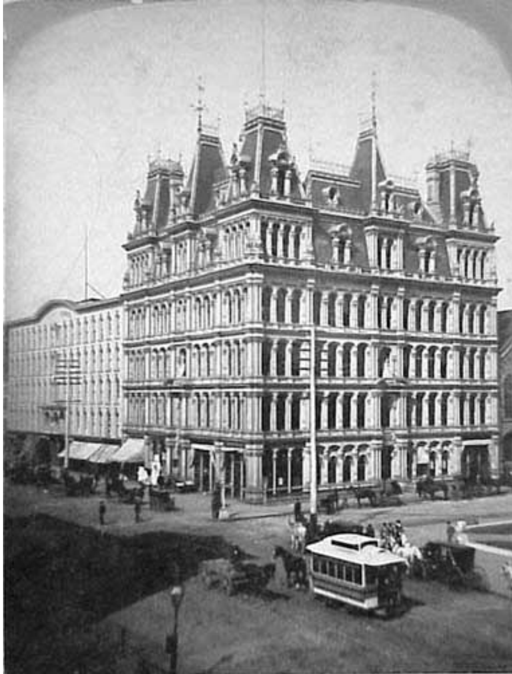
(13) The German Insurance Building, Richard A. Waite (1874-75, demolished 1957) Located at Main Street and Lafayette Square An excellent example of a Second Empire style building with a cast iron façade. Now the site of the Modernist style Tishman Building by Emory Roth & Sons (1957).
